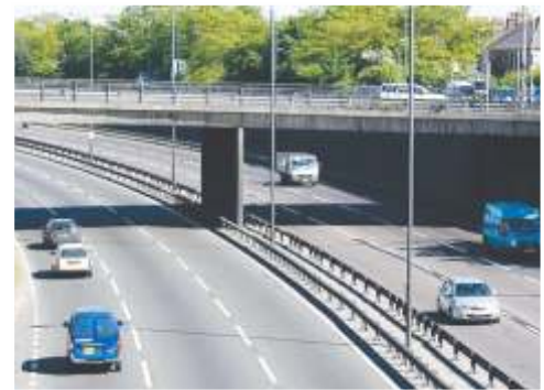
Bridge on busy road
