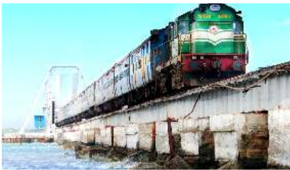
Train crossing the bridge
